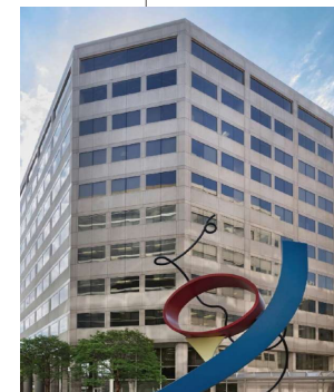
ONE UNION CENTER 810 First Street NE Washington, DC
